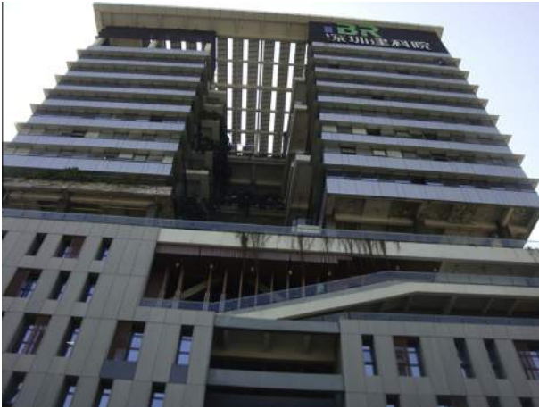
Fig. 10. Shenzhen Architecture Science Research Institute office building.
